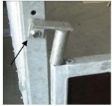
5. Secure the feed fence to the post with a M10 x 140mm screw. This will also block the pipe inside the post.
